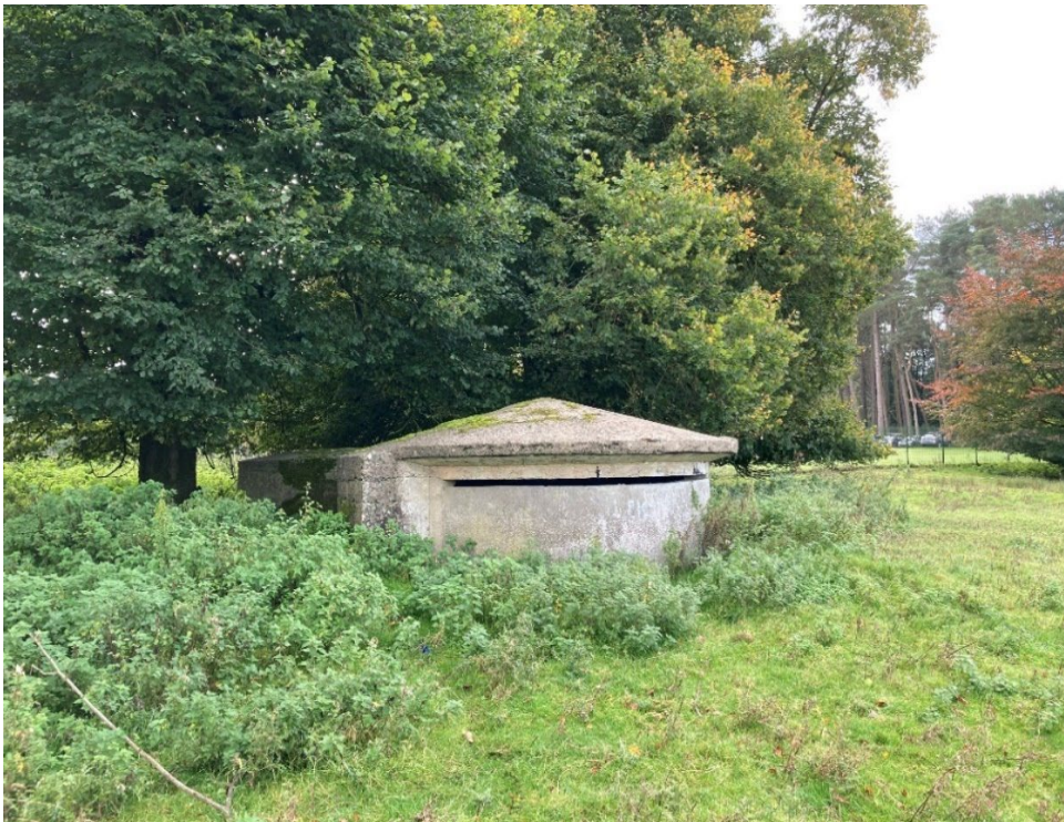
Plate 24 - Pillbox to immediate north of the Curragh Camp (Source: Research and Dig, 2021)
